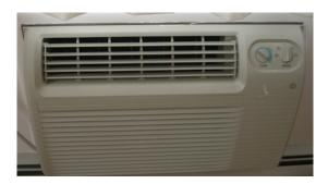
Air conditioners are most efficient when their filters are clean. This means better air flow, cleaner air, less energy and expense. If your air conditioners look like this one, then they have filters, which need to be cleaned every month or so. The frequency depends on whether you have pets that shed and other factors.
